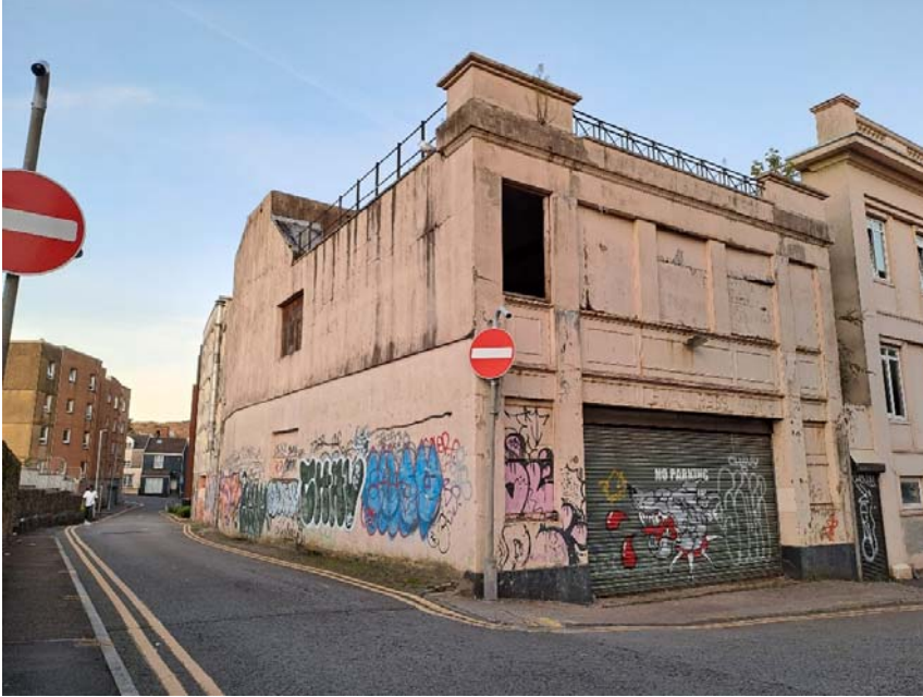
Plate 1 Surveyor View Of North West Corner (Garage Building)
