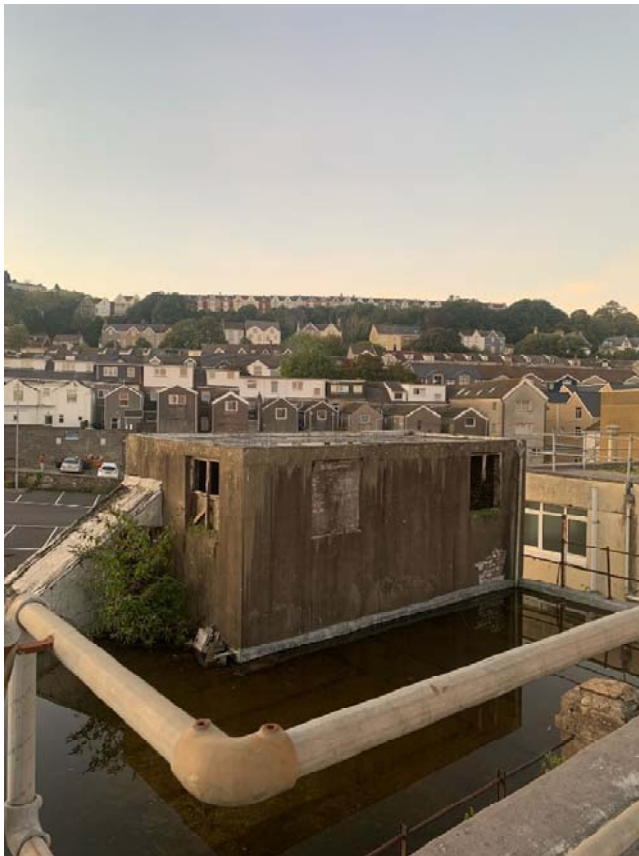
Plate 2 Surveyor View Of Roof-Top Structure To Garage Building
