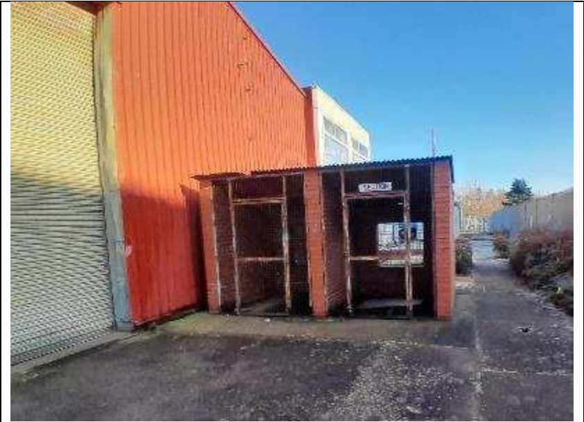
Figure 21 - exterior of B3.
