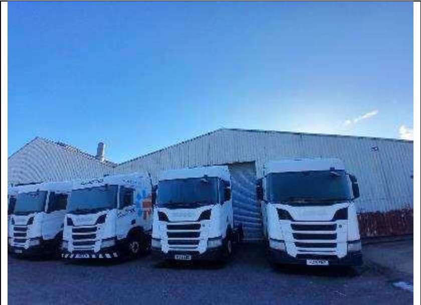
Figure 15- B1 consists of a working factory.
