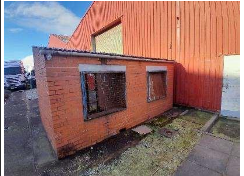
Figure 22 - exterior of B3.
