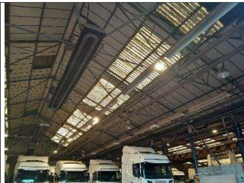
Figure 17 - interior of the factory section of B1.
