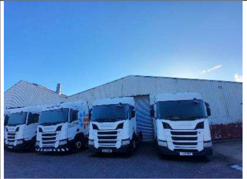
Figure 15- B1 consists of a working factory.
