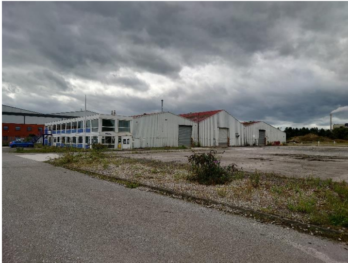
Fig.9. Existing unit (to be demolished under App Ref: 064151).
