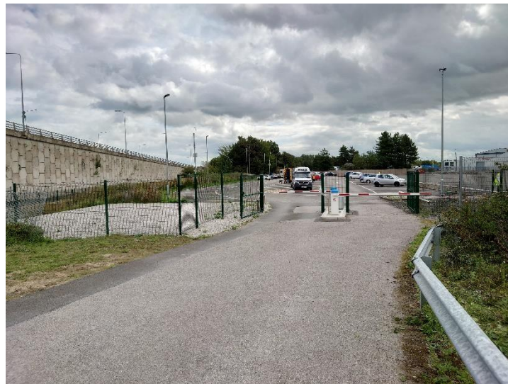
Fig.11. Existing Car Park Entrance towards the Northern Boundary.
