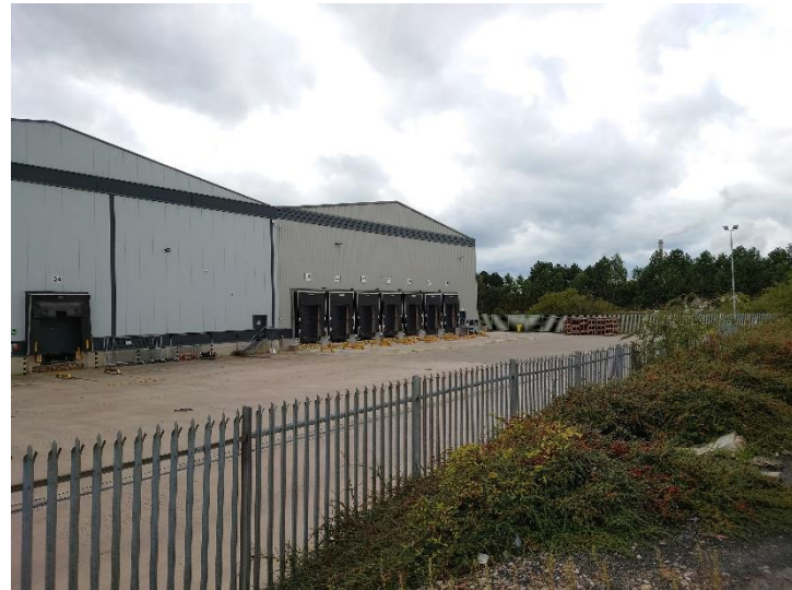
Fig.8 Fencing to Southern boundary
