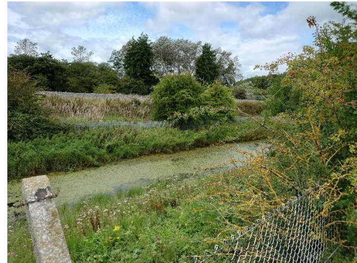
Fig 4. Existing fence towards NR Track and Land Drain.
