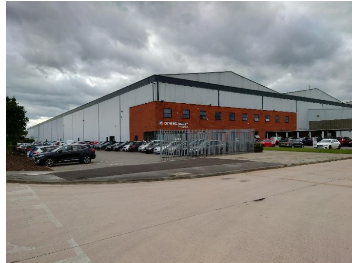
Fig 14. Existing Offices to existing distribution unit.
