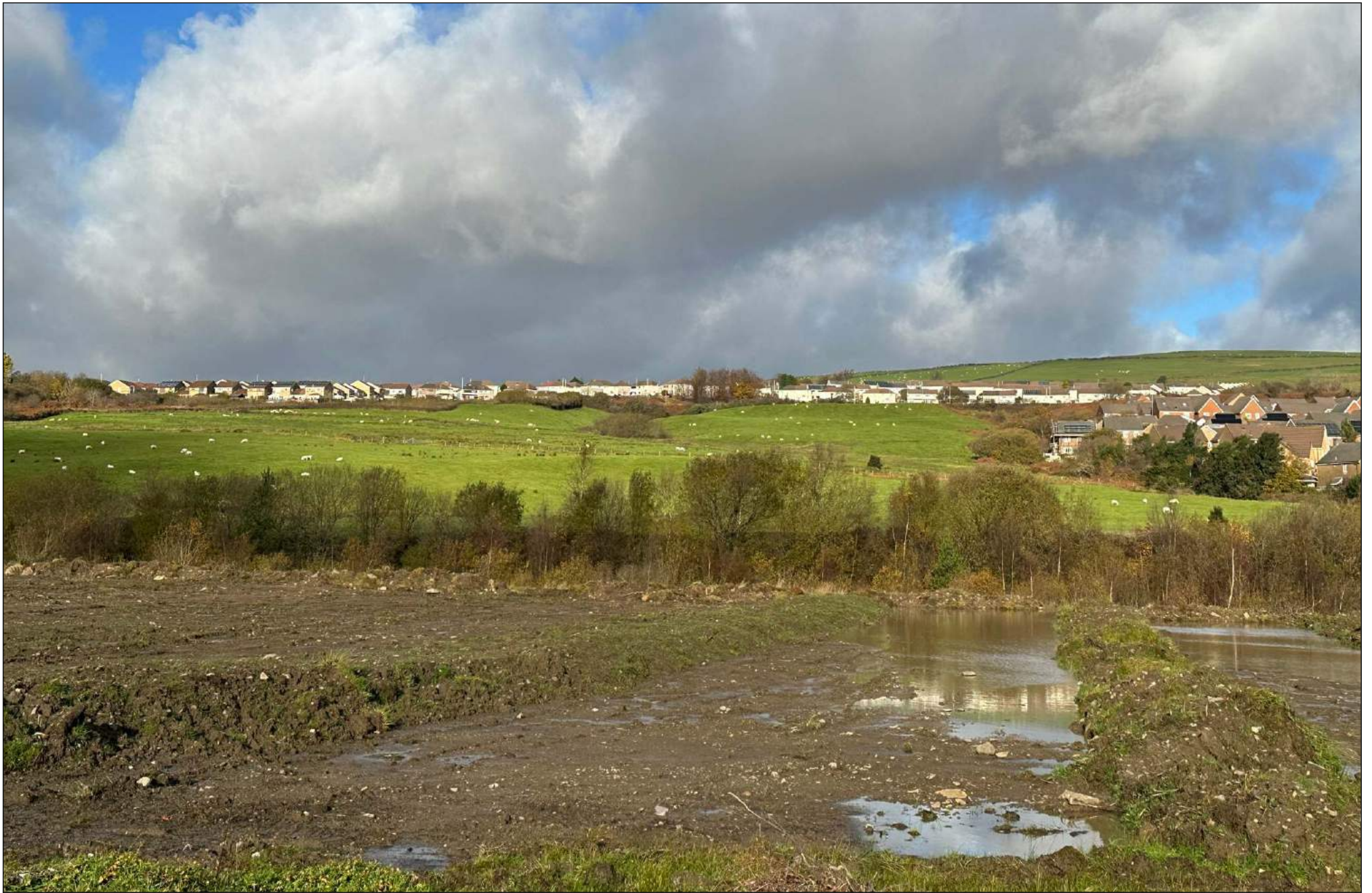
FIGURE 10 THE SITE AT PRESENT. WATER IS HOLDING ON THE SURFACE
