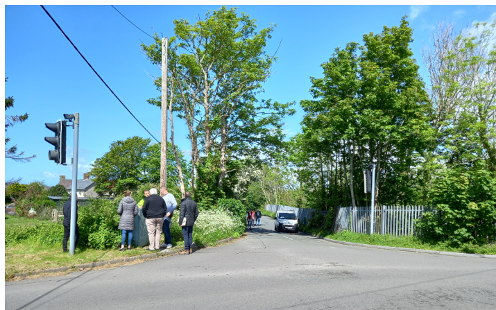
Potential Widening of Signalised Junction
